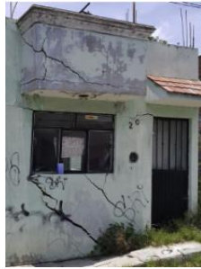
House fissuring and cracking (FIGUEROA-MIRANDA et al. 2018)
