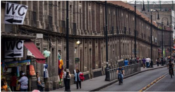
Unlevel sinking and undulating rooflines (www.sciencemag.org)
